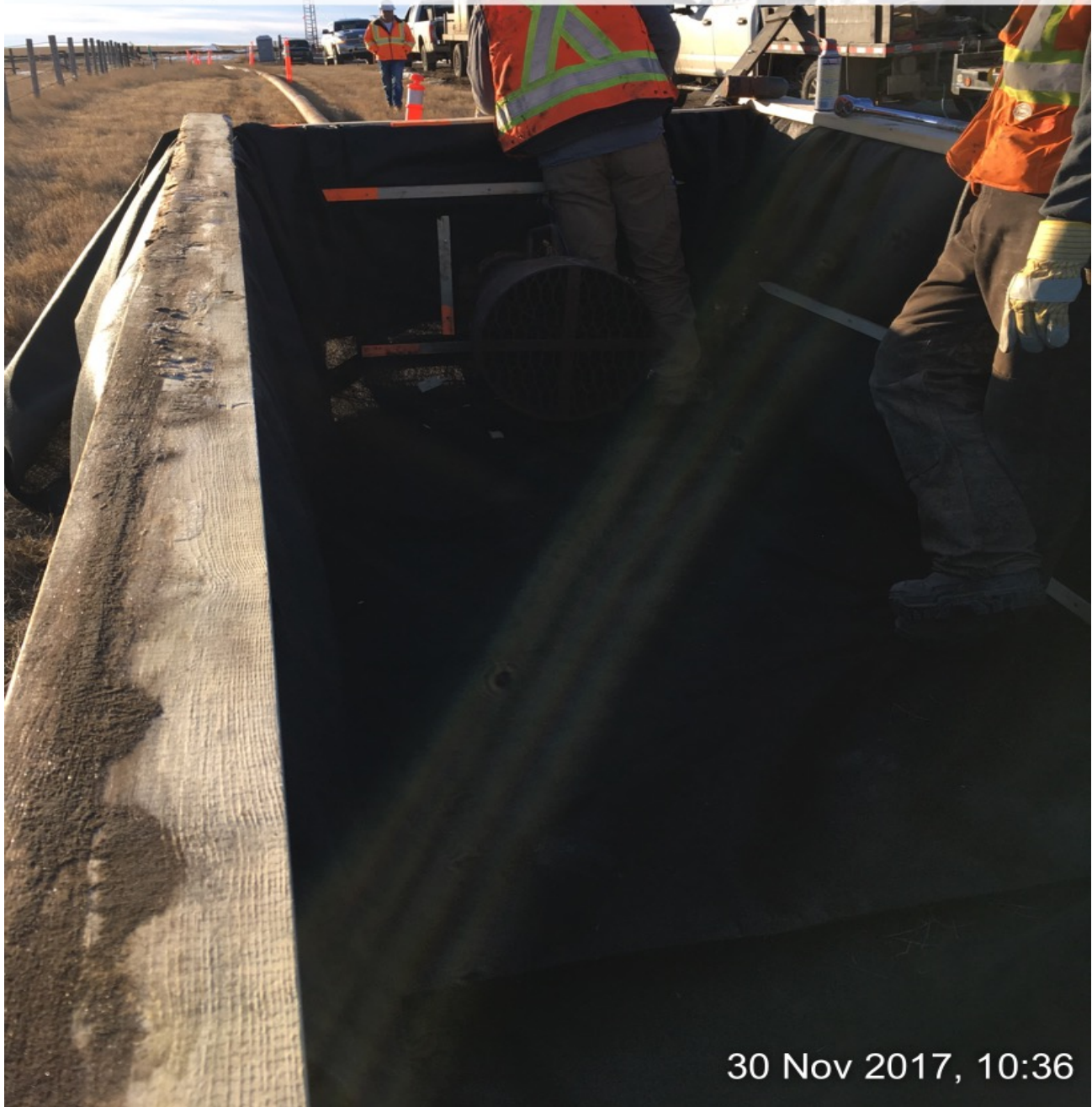
FILTERING BOX FOR DE-WATERING
