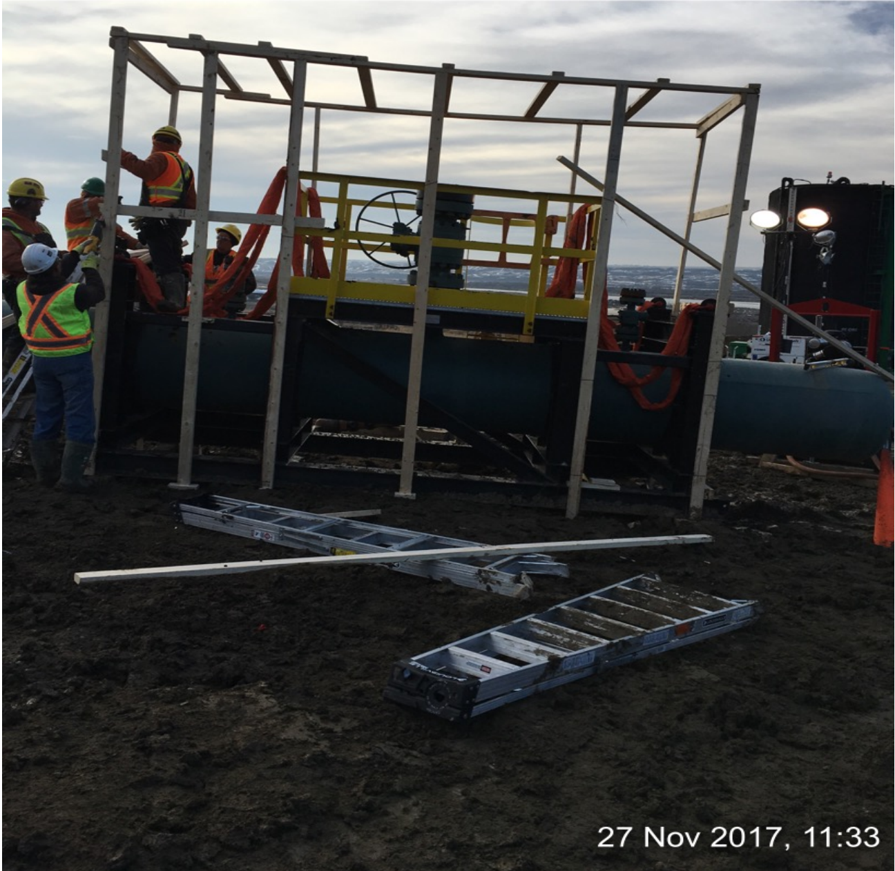
FRAMING HOARDING OVER A TEST HEAD
