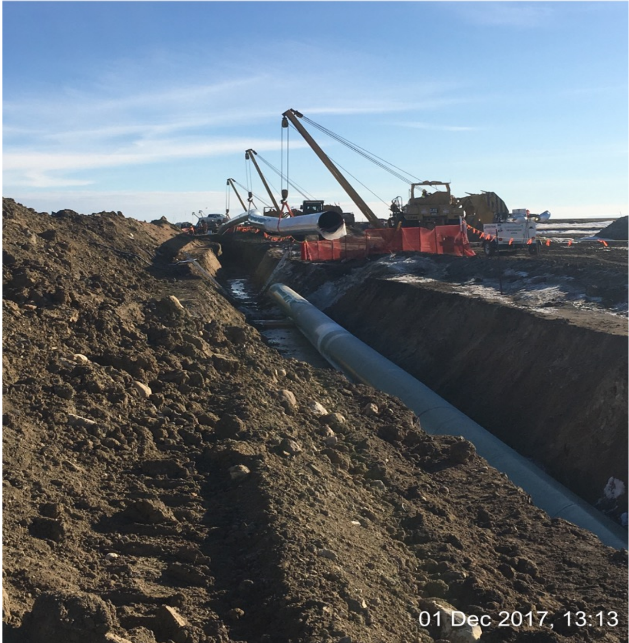
LOWERING IN SECTION OF PIPE FOR TIE IN
