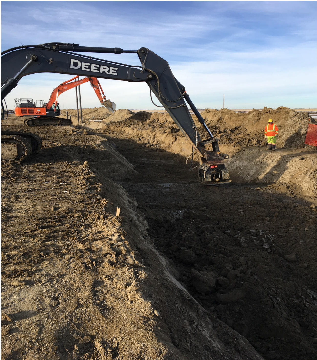
PACKING IN DIRT IN A BELL HOLE (BACKFILLING AND COMPACTION)
